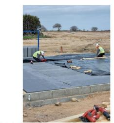
Photo 1 – Membrane works underway at the initial flatted blocks
