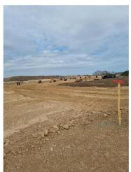
Photo 5 – Road formation with foul and surface manhole cylinders visible in the distance
