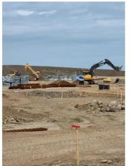
Photo 4 – Structural fill platforms being upfilled
