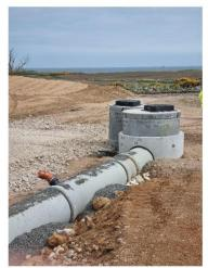
Photo 7 – Main drainage installed with typical connection visible at the pipe
